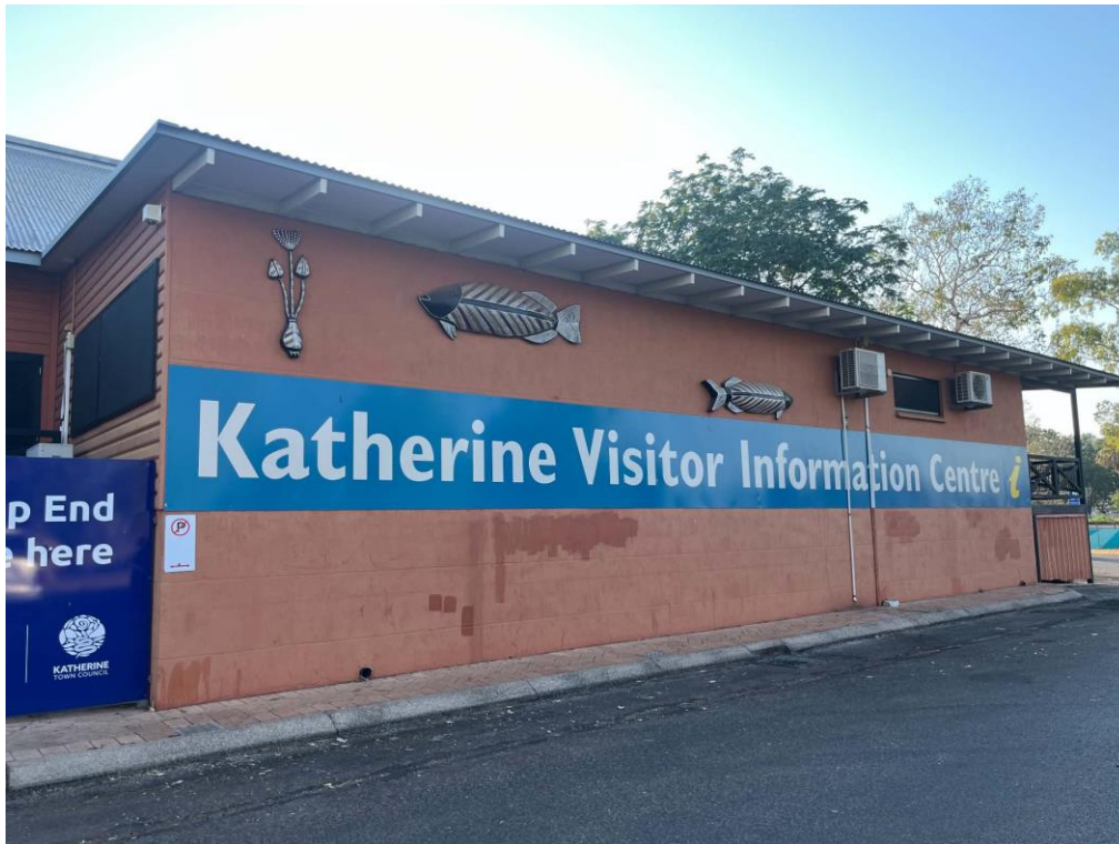
Figure 1 West Facing Wall - Katherine Visitor Information Centre
