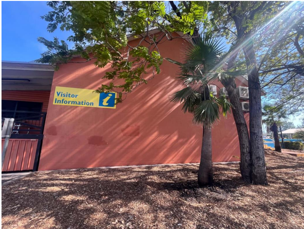
Figure 2 South Facing Wall Katherine Visitor Information Centre
