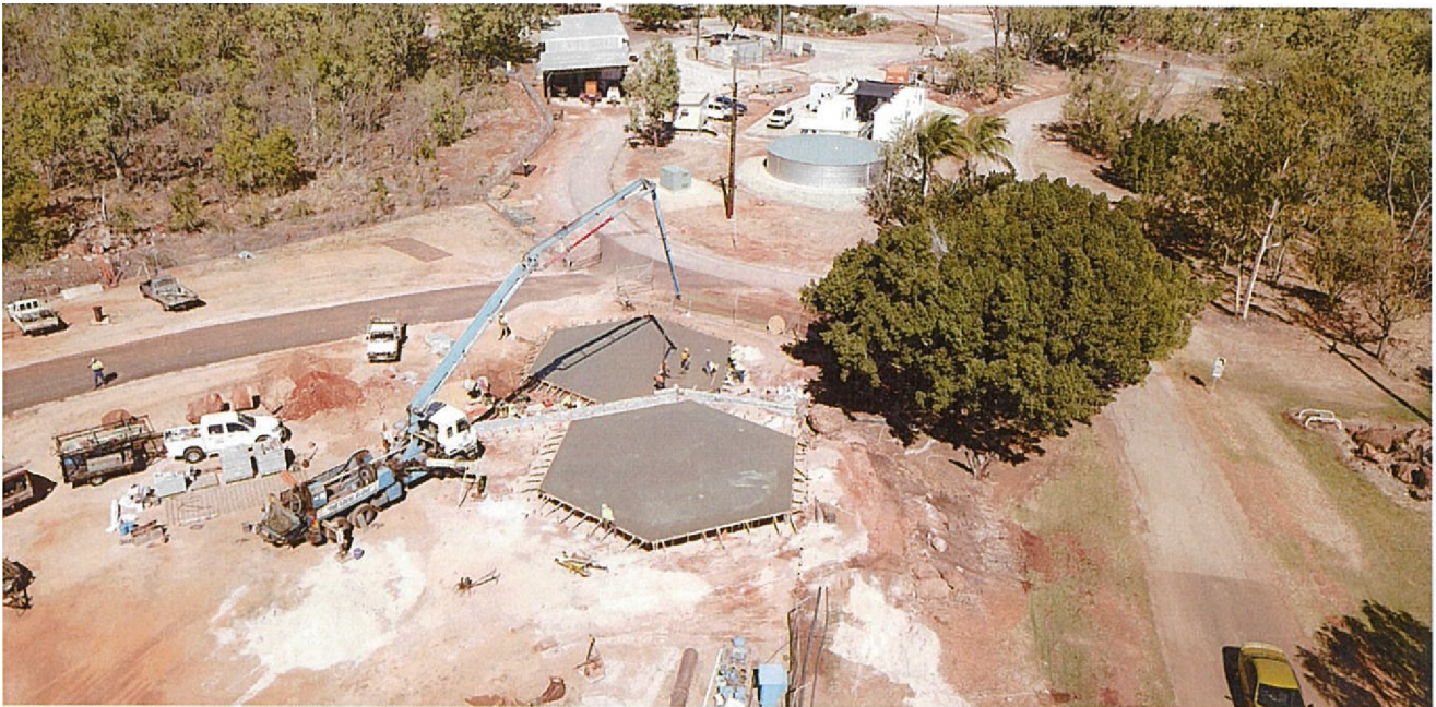
Concrete foundations for the large process tanks
