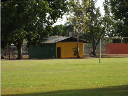
BMX/Tennis/Cricket Toilet Block
