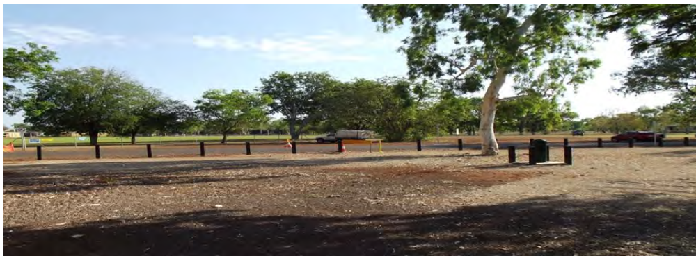
Katherine Hot Springs Top Park - Vehicle Bollards and Power Bollard
