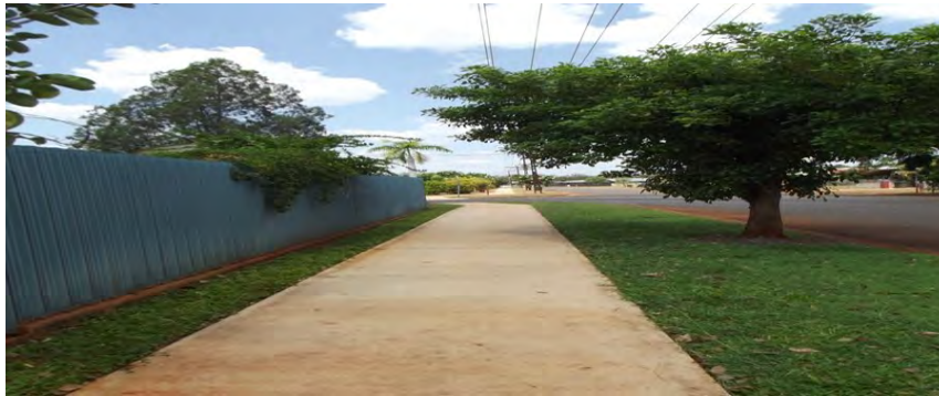
Casuarina Street Footpath Extension
