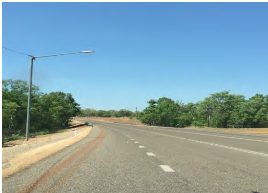
Florina Road Western Approach
