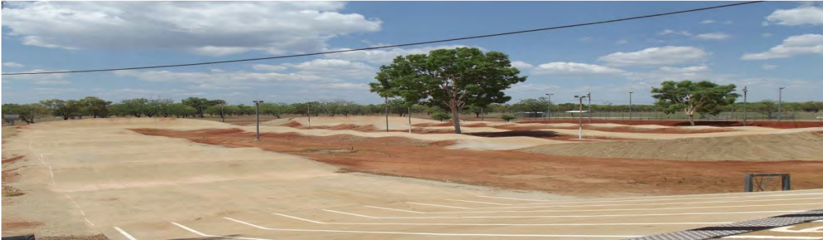
Reconstructed BMX Track & Erosion Control Berms (KCPP)
