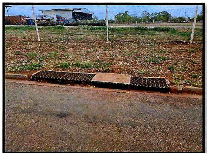
Concrete SEP drains replaced with metal grates
