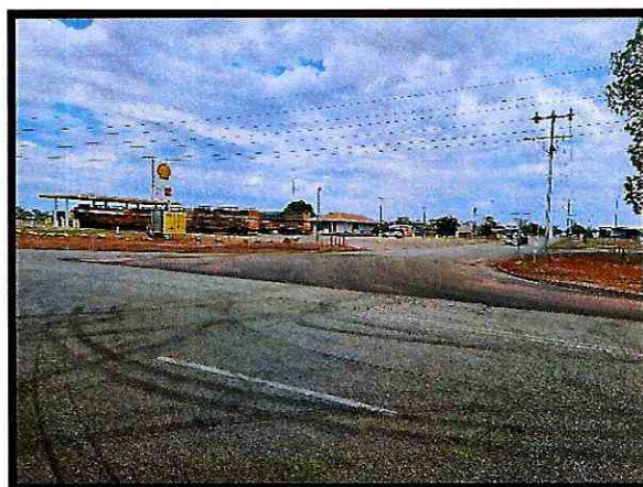
End result of works on Gillard Street
