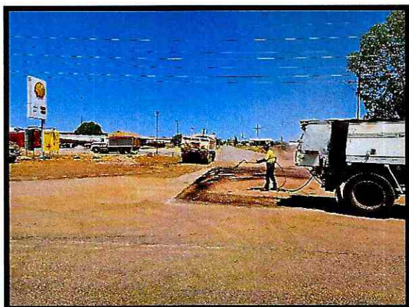
Contractor carrying out works on Gillard Street
