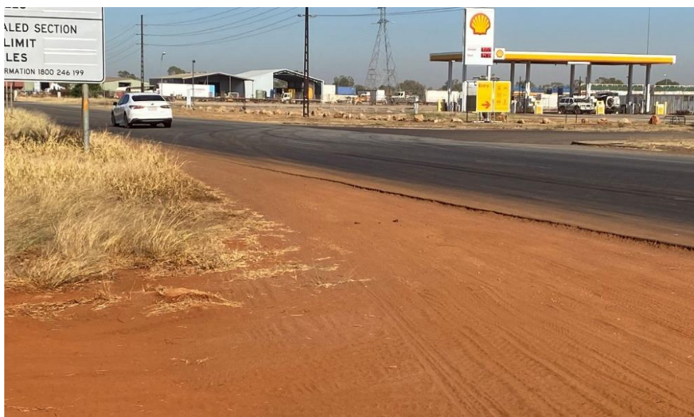
Zimin Drive shoulder drop off (above) and remediation works (below)
