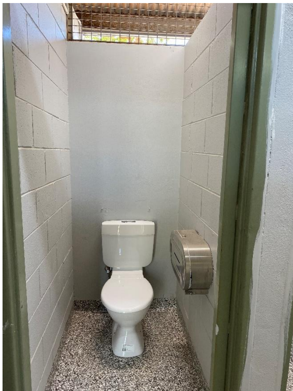
New epoxy flooring and toilet fittings
