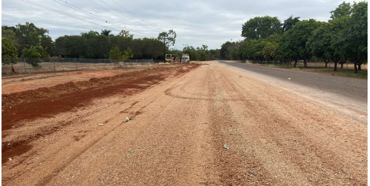
Morris Road remediation works
