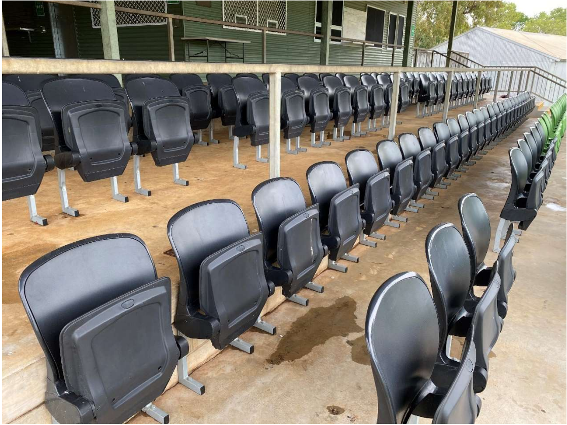
Pressure cleaning of Grandstand for Katherine Annual Show
