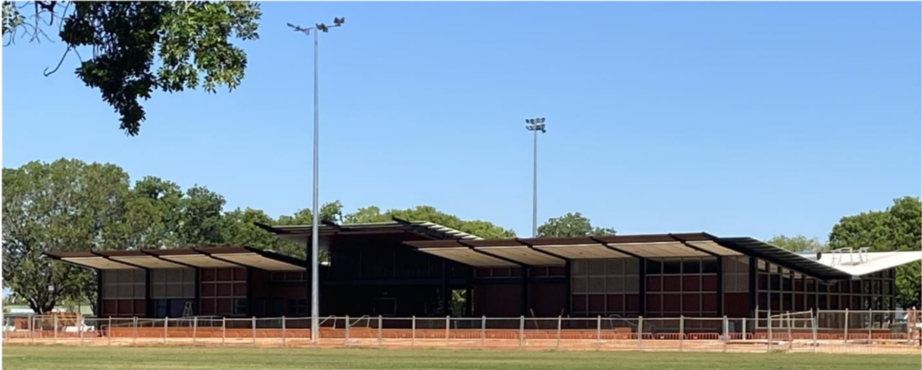
Framework and Facades in Progress
