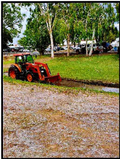
KTC Staff clearing of the drain - BEFORE
