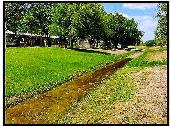
AFTER clearing of the drain
