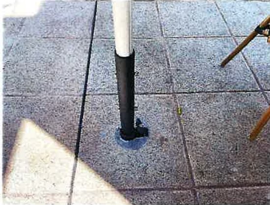
Flush mount umbrella stand holders installed in Town Square
