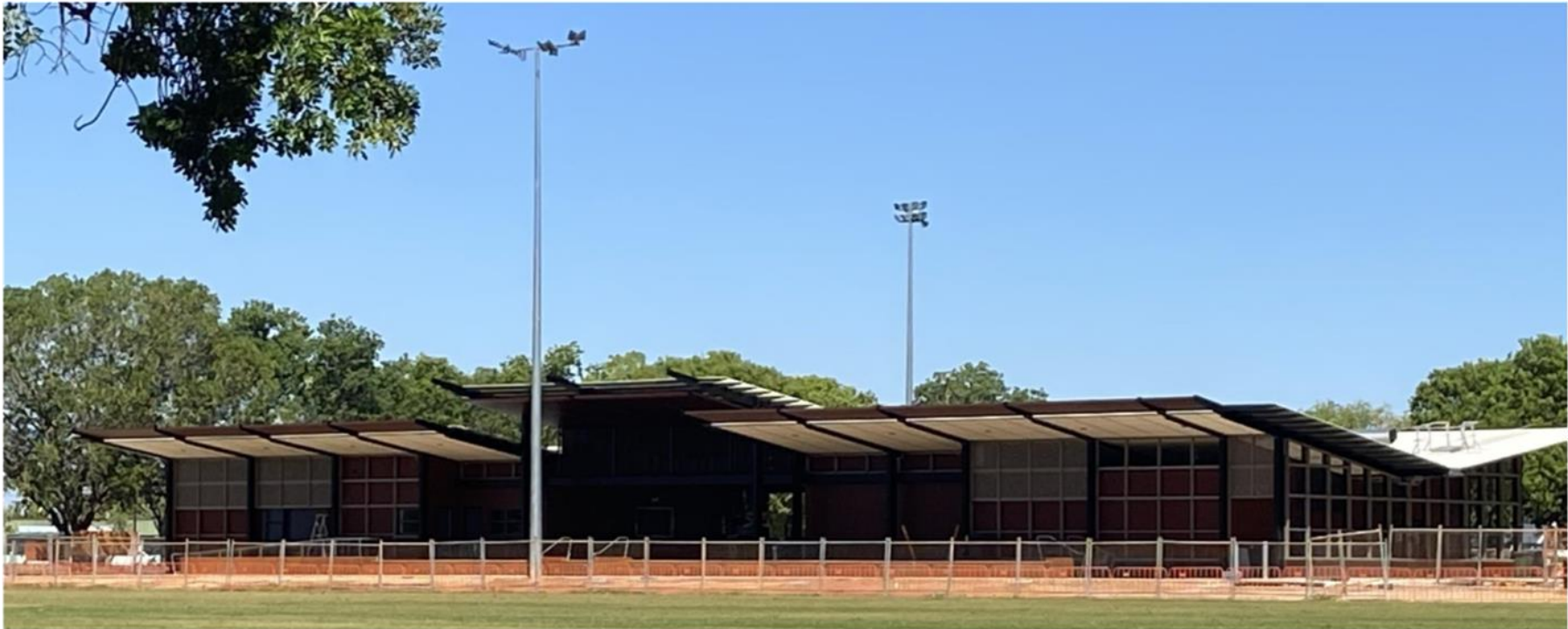
Framework and Facades in Progress
