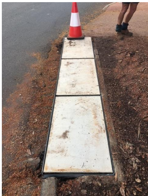
Pit cover replacement First Street
