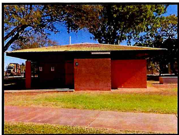
Ryan Park Toilets Before
