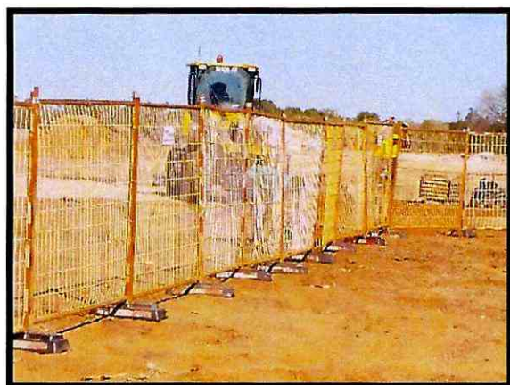
Waste Transfer staff erecting the exclusion zone temporary fencing
