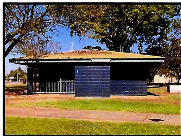
Ryan Park Toilets After (roof works scheduled for August)
