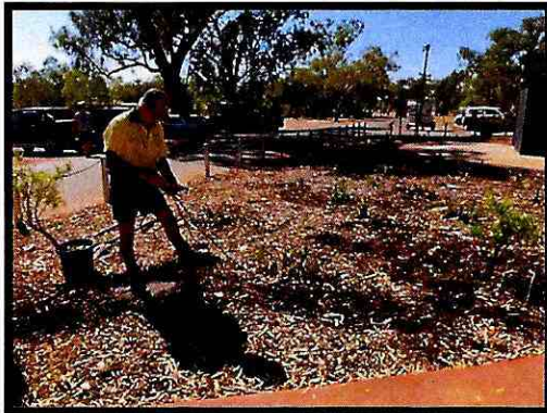
KTC staff installing irrigation at the Hot Springs
