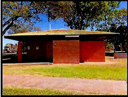
Ryan Park toilets before
