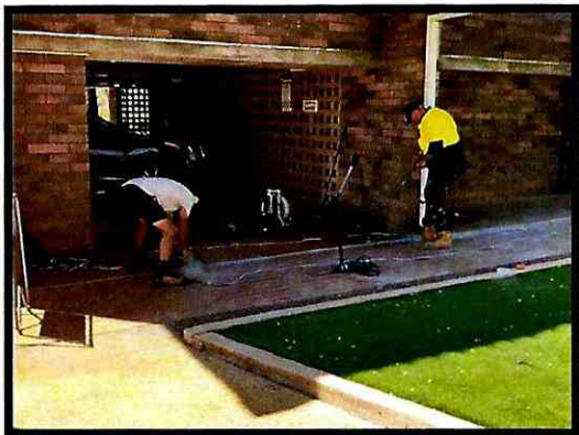
KTC staff preparing the surface for pebblecrete at the Civic Centre
