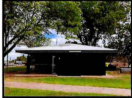
Ryan Park toilets completed
